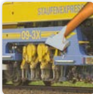
14 - Rail track construction
