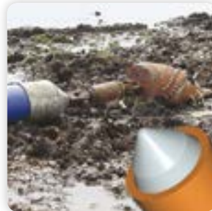
7 - Horizontal directional drilling HDD
